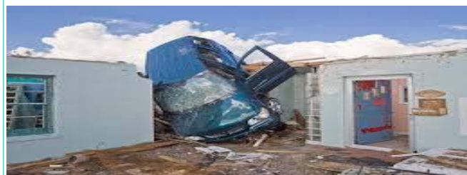
Figure 5: Damage caused by Tornadoes.
