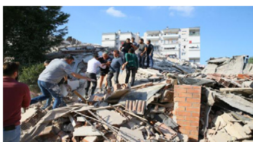
Figure 15: Earthquake caused structural damage.
